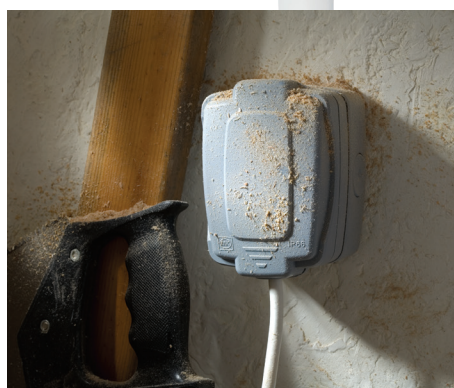
DUST PROOF CONNECTION TO SAFEGUARD WORK AREAS.
