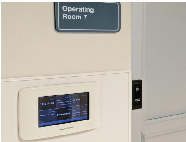
To ensure these cutting-edge ORs are fully compliant with healthcare specifications, the Surgery Center's facilities team sought to replace vintage variable air volume (VAV) boxes with an easier to control, more consistent airflow management system.
