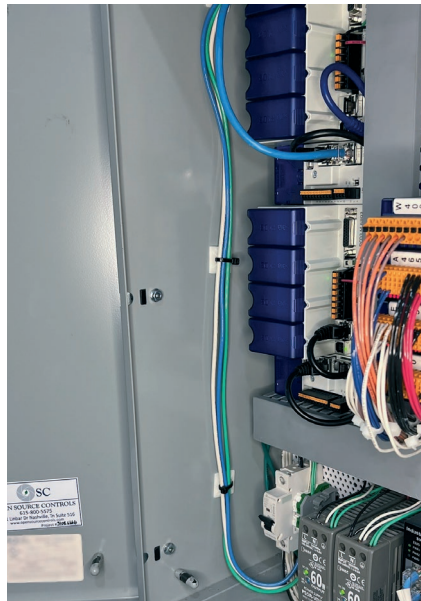
Control panel for data server cooling control. Redundancy controller for zero downtime.
