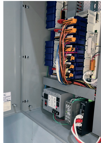
Air handling control with redundancy to provide control for optimal operating temperatures for the servers.
