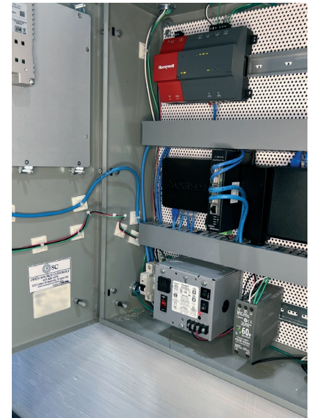
Using Jace to tie the system together and provide a seamless GUI for the customer.
